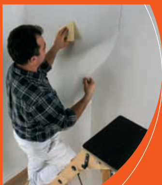
2 - Apply the wall covering, smooth it and cut off the excess
