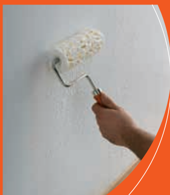
1 - Apply the vinyl glue on the wall evenly by means of roller
