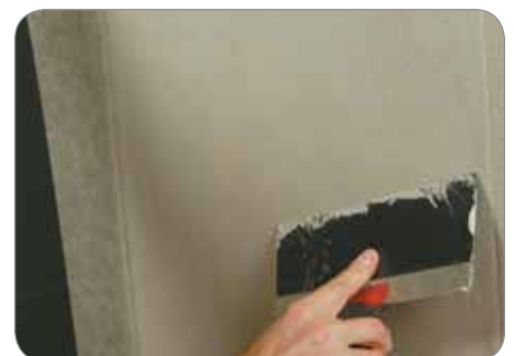
Wall reinforcement
