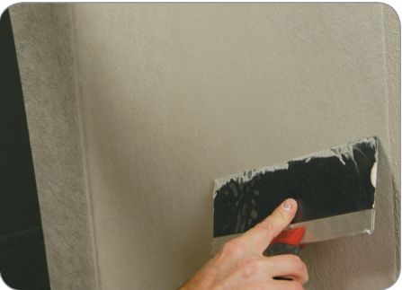
Wall reinforcement
